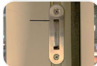
**LINE UP THE BOTTOM KEEPER ALLOWING 1/8 INCH GAP FROM YOUR LINE TO THE TOP & MARK THE HOLES.**
