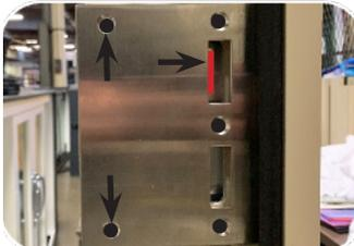
**LINE UP WITH THE TOP LINE AND SLIDE BACK SO THE DEADBOLT SLOT IS FLUSH WITH THE EXTERIOR EDGE OF THE CUT OUT HOLE. MARK THE HOLES FOR THE SCREWS.**
