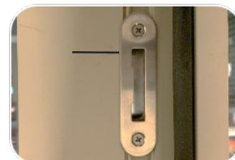
**SECURE THE HOOK KEEPER TO THE JAMB.**
