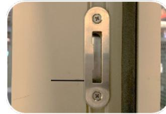
**SECURE THE HOOK KEEPER TO THE JAMB.**
